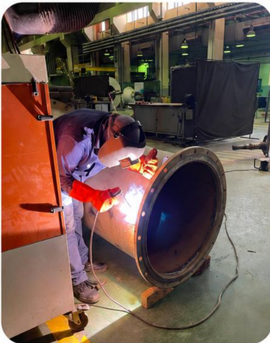
Onsite Welding & Fabrication service.
