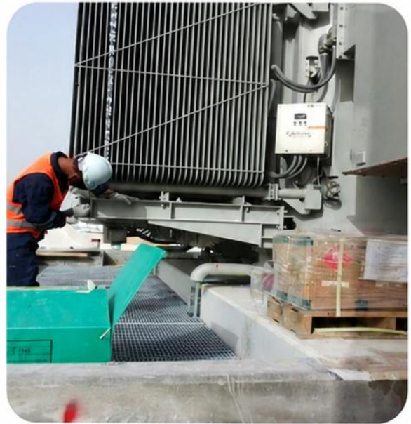
Maintenance & Repair of Transformer & Cooling Fans.
