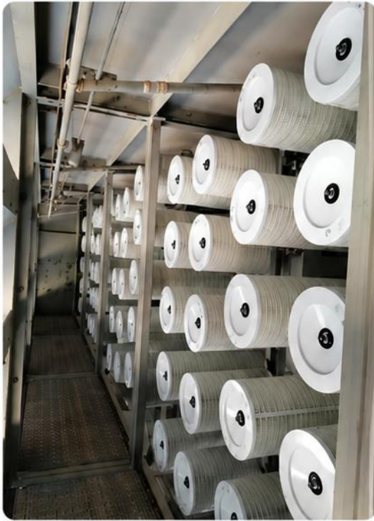
Gas Turbine Inlet Filter replacement & alignment. Replacement of pulsating header and solenoid valves.
